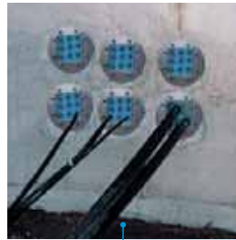
Transits into foundation.
