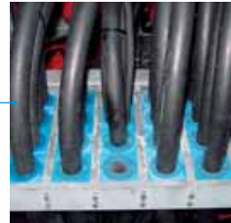
Retention systems below nacelle and in tower.
