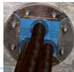
Transits for foundations.
