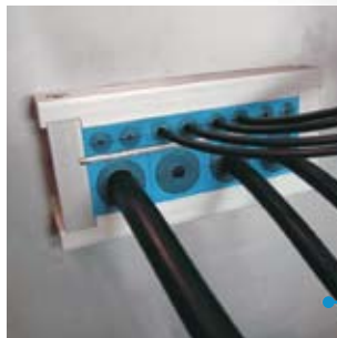
The Roxtec CF 24 transit simplifies installation around existing cables. Here, installed in the wall of a power drive.
